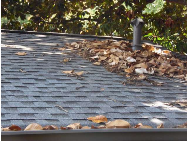
Roof Close Up Rec No. 2019-09-02
