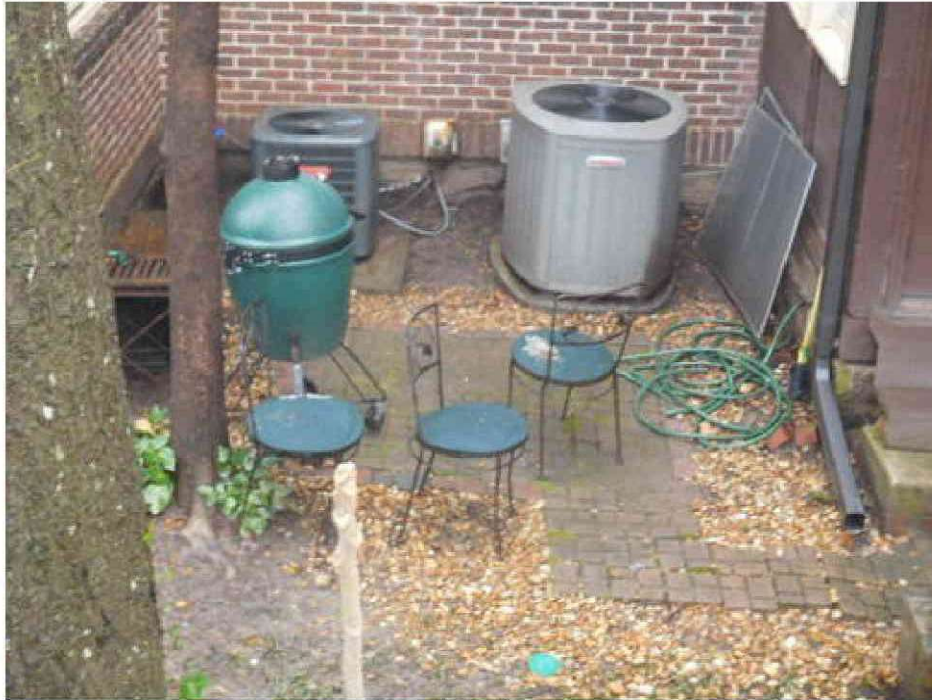
Grill within 10' of Bldg. 1021
